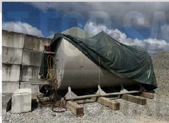
KPDN photo shows the skid tank at the raided premises found to contain the diesel.
